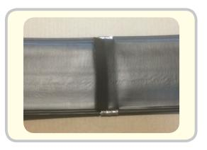
Remove any excess centre panel with a pair of snips (or knife). Then flatten the centre panel out to cover the gap.
