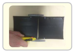
2 Bend the centre panel out of the way and then use our wire strippers to remove the plastic from the wire (similar to rail preparation for attachment to the end post). Repeat for all 4 wires to be joined.
